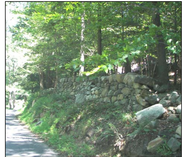
Stonewall along Hunterbrook Road, Hunterbrook.
