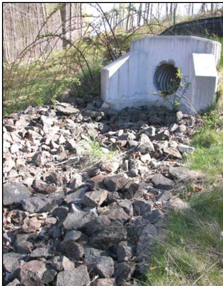
A drainage outfall.
