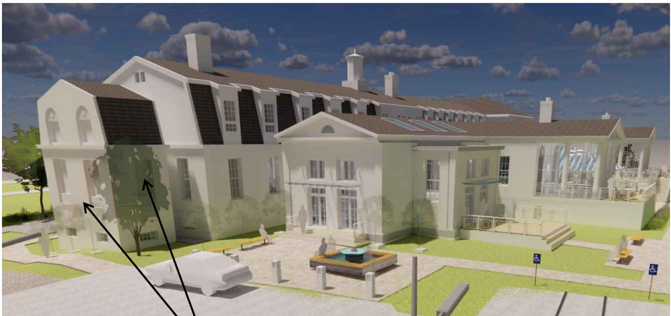
New 2 Story HVAC Tower w/ Generator & HP Condensing Units
