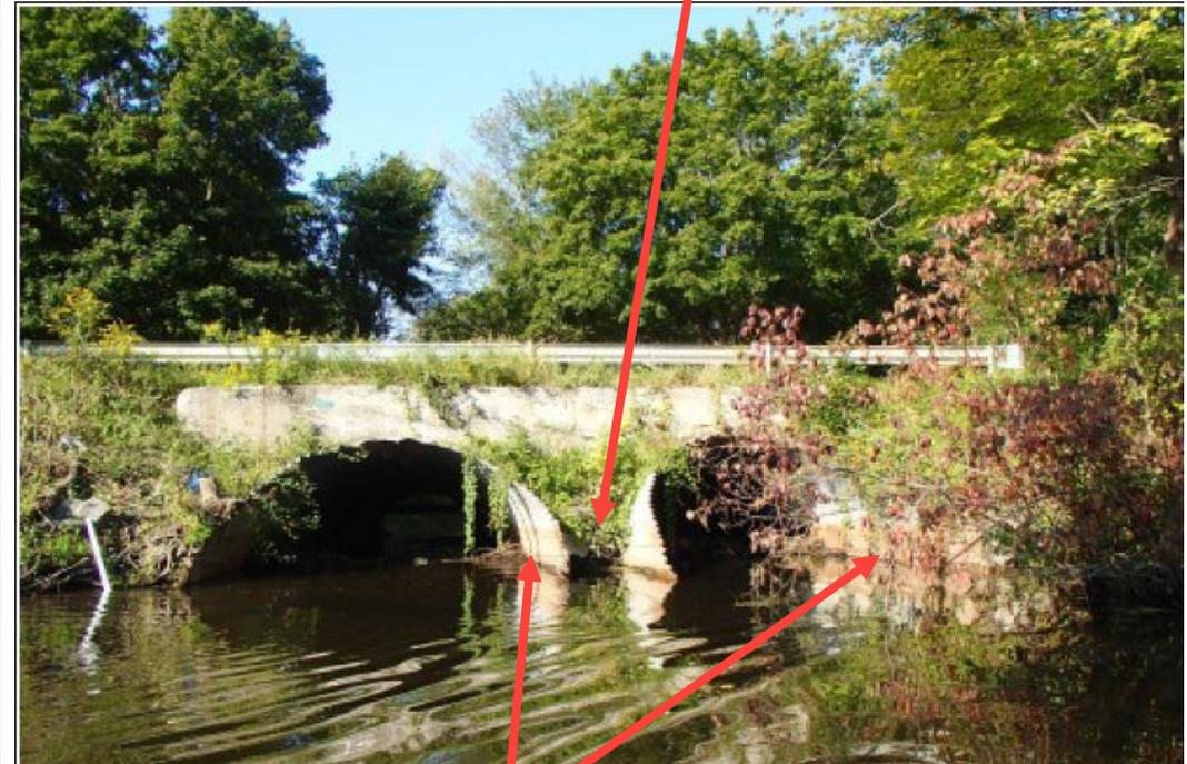
Significant corrosion and section loss of barrels – Yellow Flag Condition
