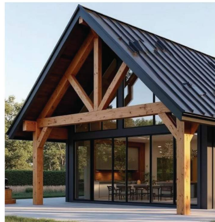
6. Heavy Timber Framing
