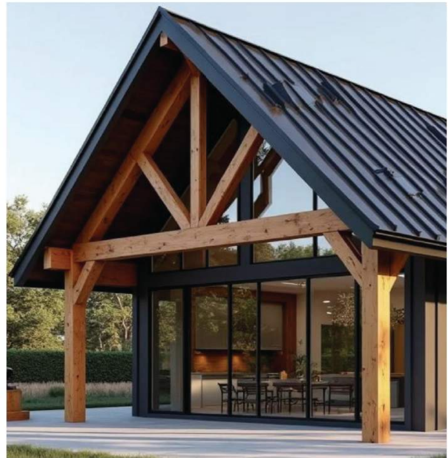
6. Heavy Timber Framing
