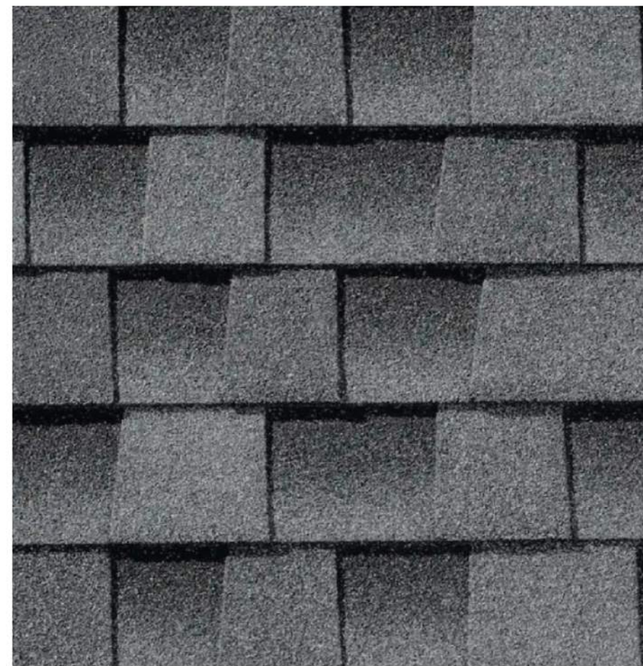
5. Asphalt Shingle Roof
