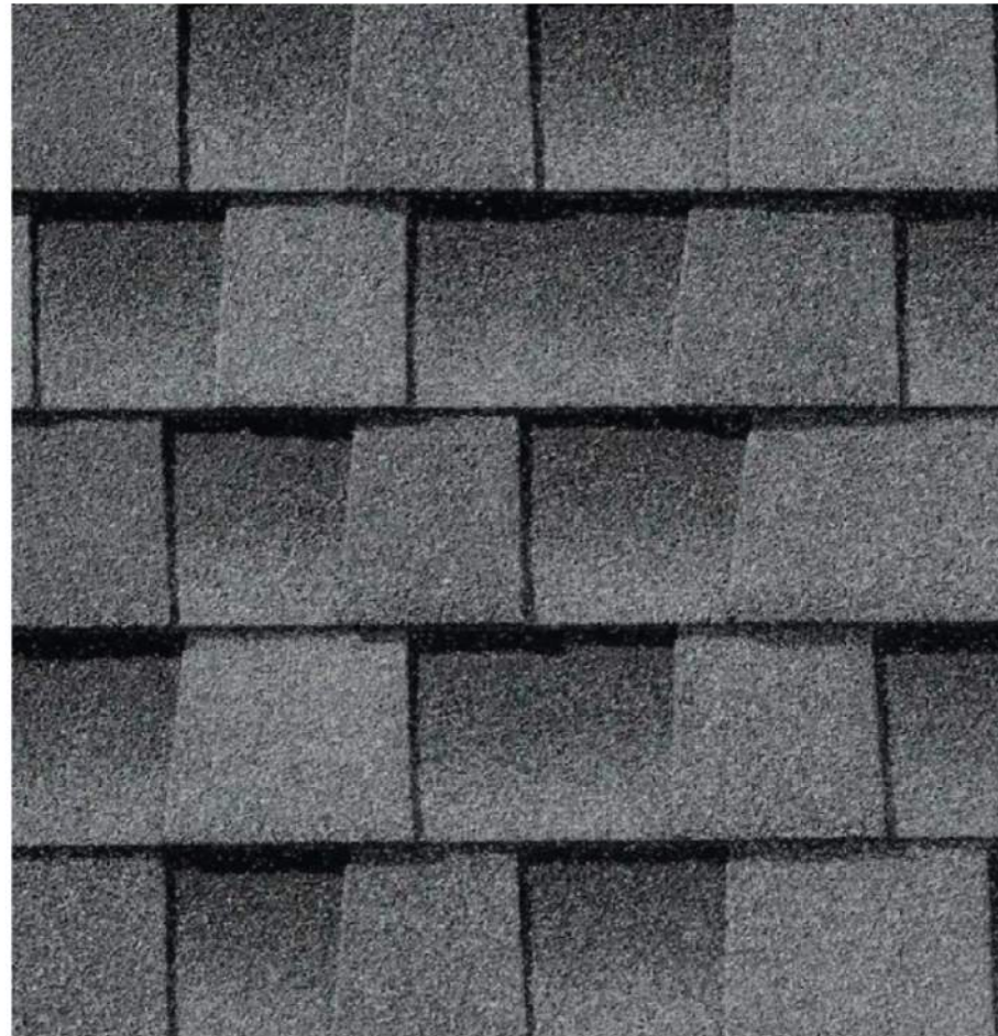
5. Asphalt Shingle Roof
