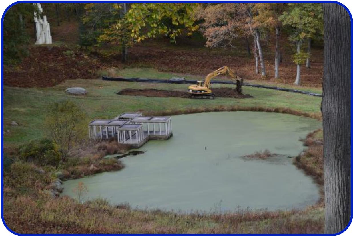
Flat "pad" being built for 120' x 30' dewatering bag (geotextile tube)
